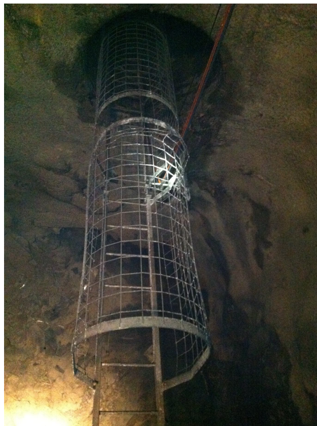
An escape way between levels
