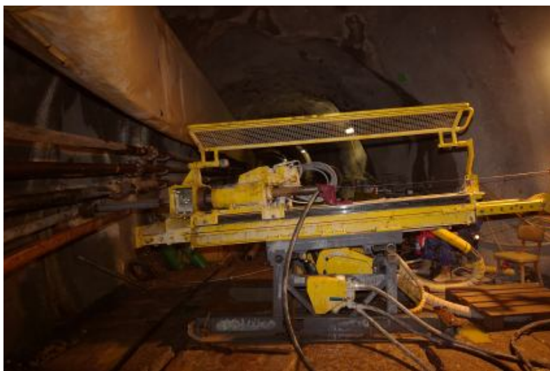
Scaling is always required around a diamond drill rig
