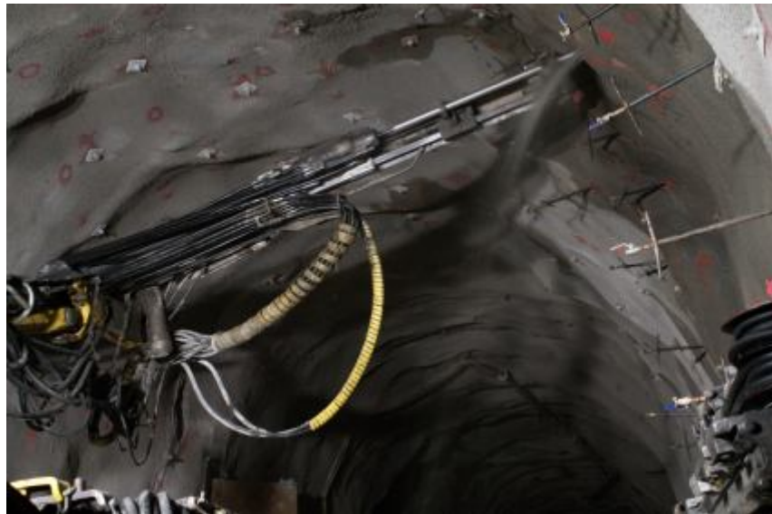
Twin Boom Jumbo installing the Ground support through shotcrete
