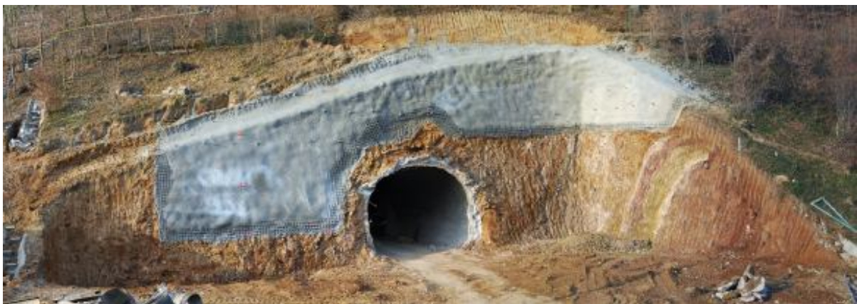
The portal to the underground mine
