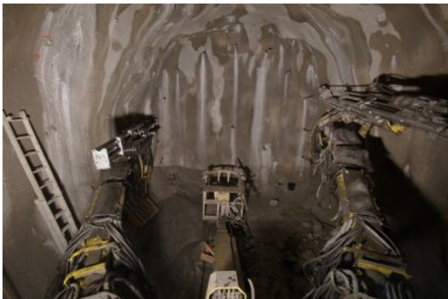
A Twin Boom Jumbo boring the face
